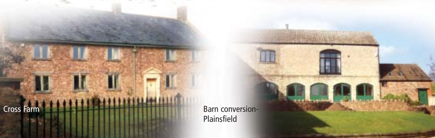
Before and after restoration: glazed porch removed, period windows and door reinstated; paint removed from stonework.
