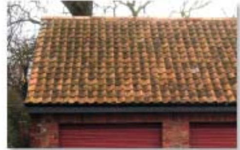
Pantiles on modern garage of traditional construction.
