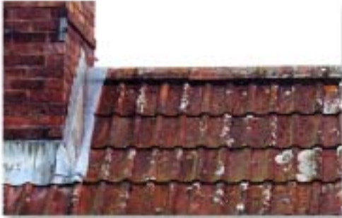
Double Roman tiles on an old cottage
