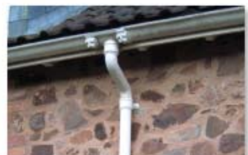
Cast iron gutter and downpipe..
