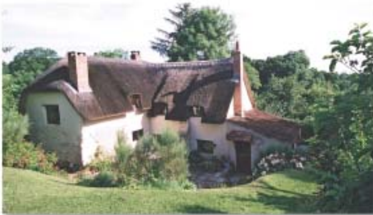
Thatched cob cottage destroyed by fire restored to original form.
