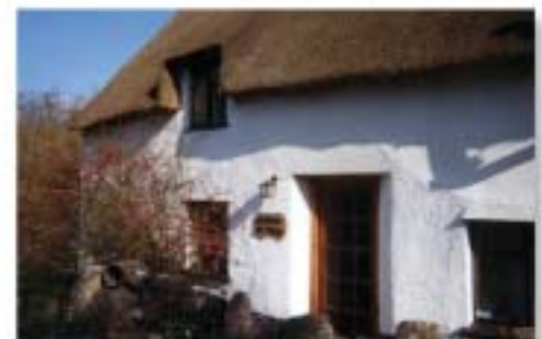
Lime based render on cob, with thatched roof
