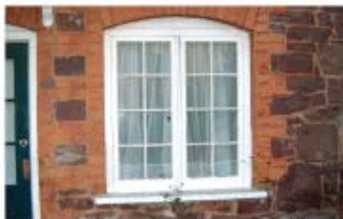
Red sandstone with brick dressings and traditional casement window.
