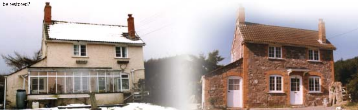
Before and after restoration: glazed porch removed, period windows and door reinstated; paint removed from stonework.
