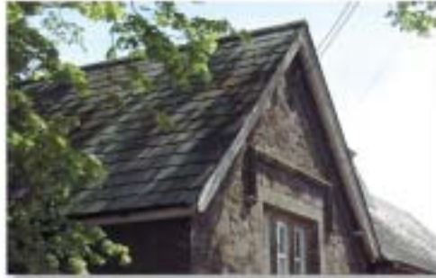
Victorian slate roofing on the village hall
