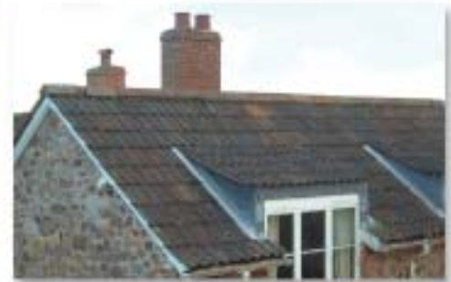
Extension with dormer and reclaimed double roman tiles
