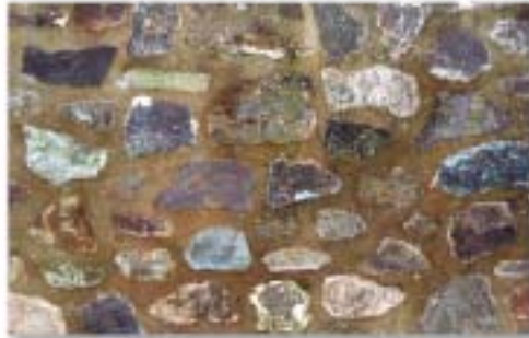
Rough hewn local sandstone / slate with flush pointing
