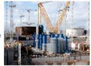
Once the concrete is poured, it will create the table upon which the turbine and turbine generator will sit.
